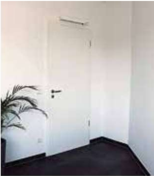
Closed The door can be opened automatically and also at any time by hand.
